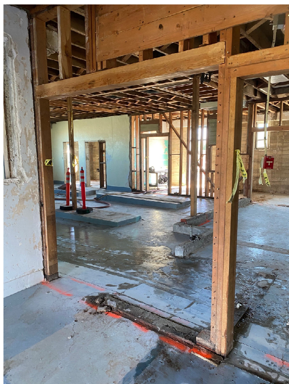
View of Locker Rm from Lobby Area
