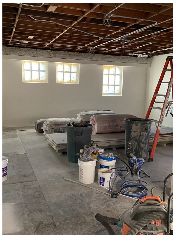
New Classroom View
